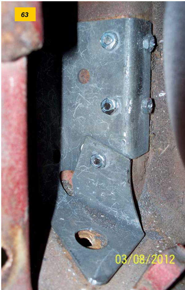
(LEFT) the inside view of those same bolts, going through the rear body mount reinforcement.
