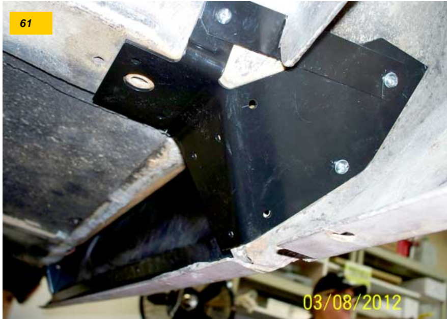
(LEFT) front view of the front body mount reinforcement in place with bolts going through the fiberglass and into the nuts we welded on the inner rocker panel support.
